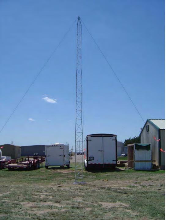
Elevations of transmitter and receiver must sum to 30' per km of path length
