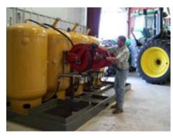
Figure 2: Portable tanks, nurse tanks, or skids (such as those provided by Sage Oil Vac, Inc. in Amarillo) are exempt from SPCC Regulations and are not counted in the total on-site fuel and oil volume. Although secondary containment is not specifically required for this class of containers, care should be taken to minimize the potential to drain fuel, oil, or waste oil into water sources. *Any such discharge event is in violation of state and federal environmental laws*.
