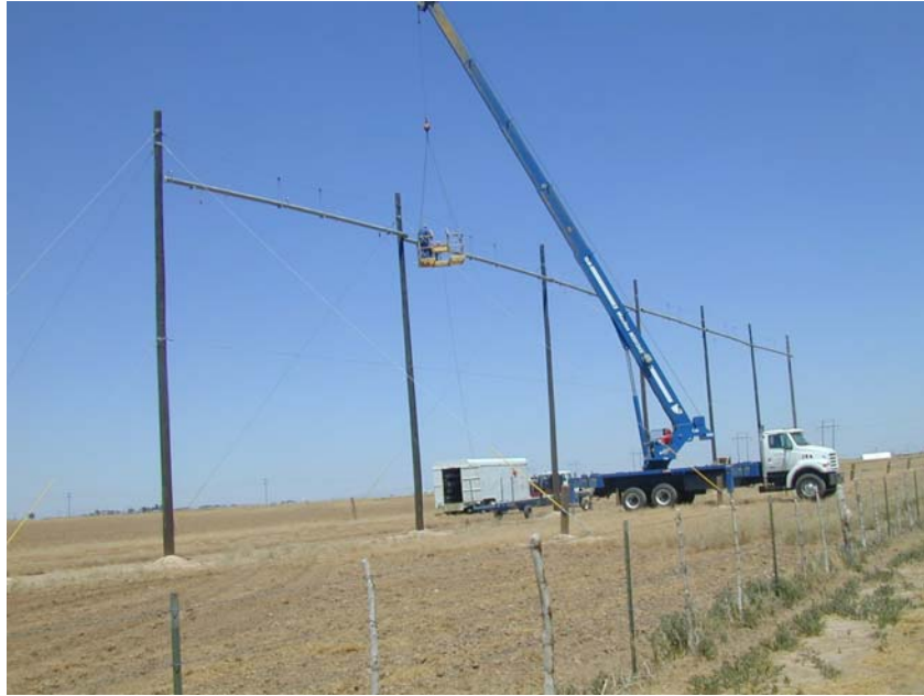
Figure 1. Contractors raising the irrigation pipe into place and attaching it to the high-tensile, braided steel cable with rolling blocks and wire slings.
